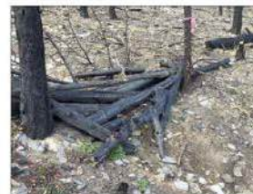
CONSTRUCTED SIMPLE LOG STRUCTURE GULLY TREATMENT PHOTO SOURCE: JN ASSOCIATES
