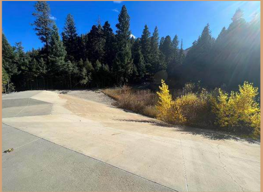
Concrete (permanent) sediment basin at the mouth of a tributary to West Monument Creek, installed following the Waldo Canyon Fire (2018). Photo: Stillwater Sciences
