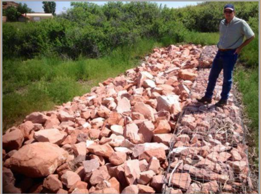
Sediment Basin in Soldier Canyon after High Park Fire (2012). This Gabion wall was quite efficient at settling out sediments while allowing water to move through. Following removal, the sediment collected was used to improve the conditions on local roads. Photo: JW Associates
