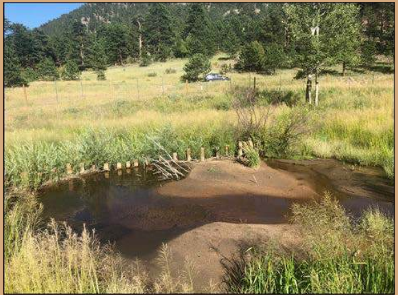
Beaver Dam Analogs installed along Fish Creek in Estes Park, have trapped sediment and reconnected the floodplain. Photo: Stillwater Sciences
