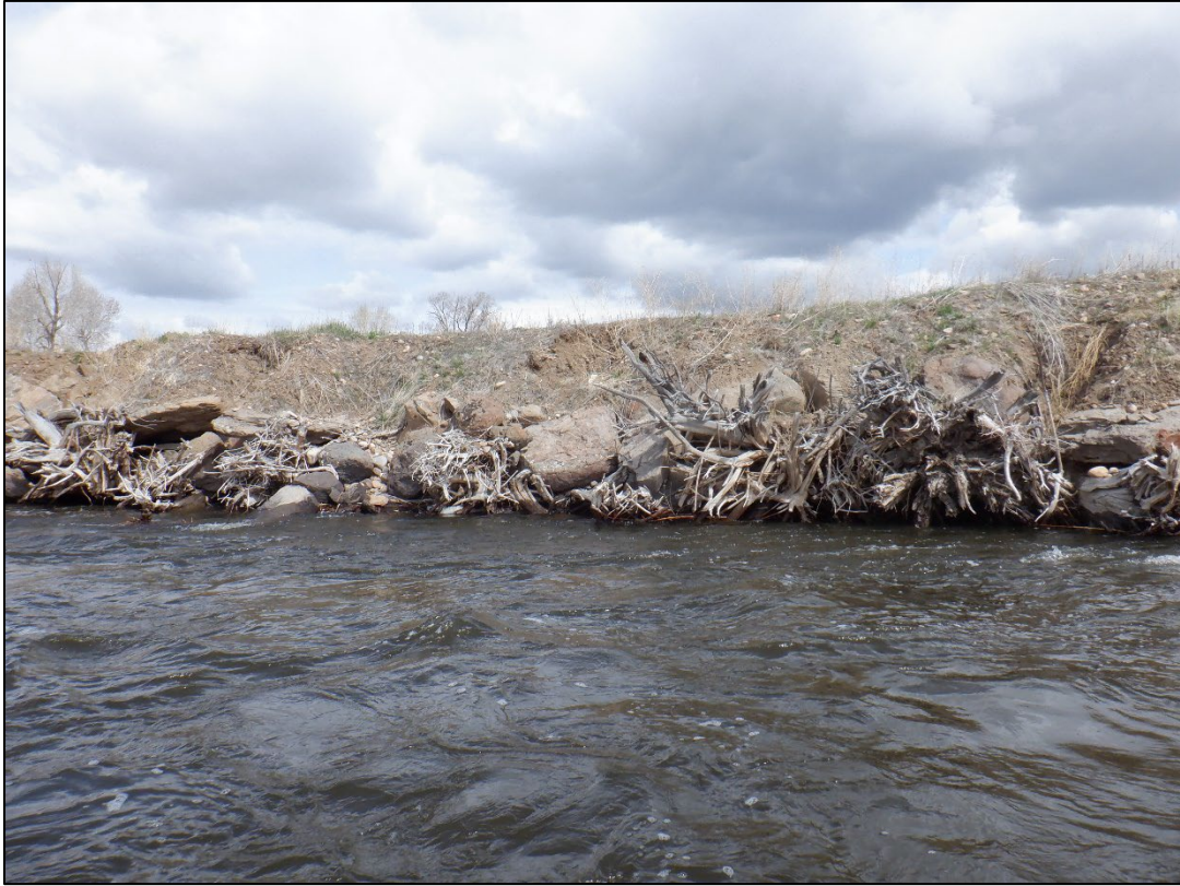
Figure A-7. Bank armoring with rootwads and large boulders.
