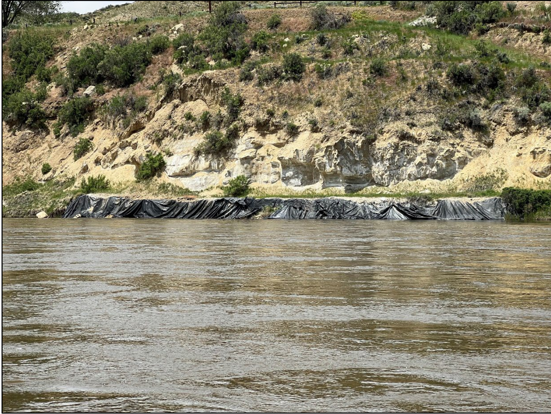
Figure A-9. Bank armoring with heavy plastic.
