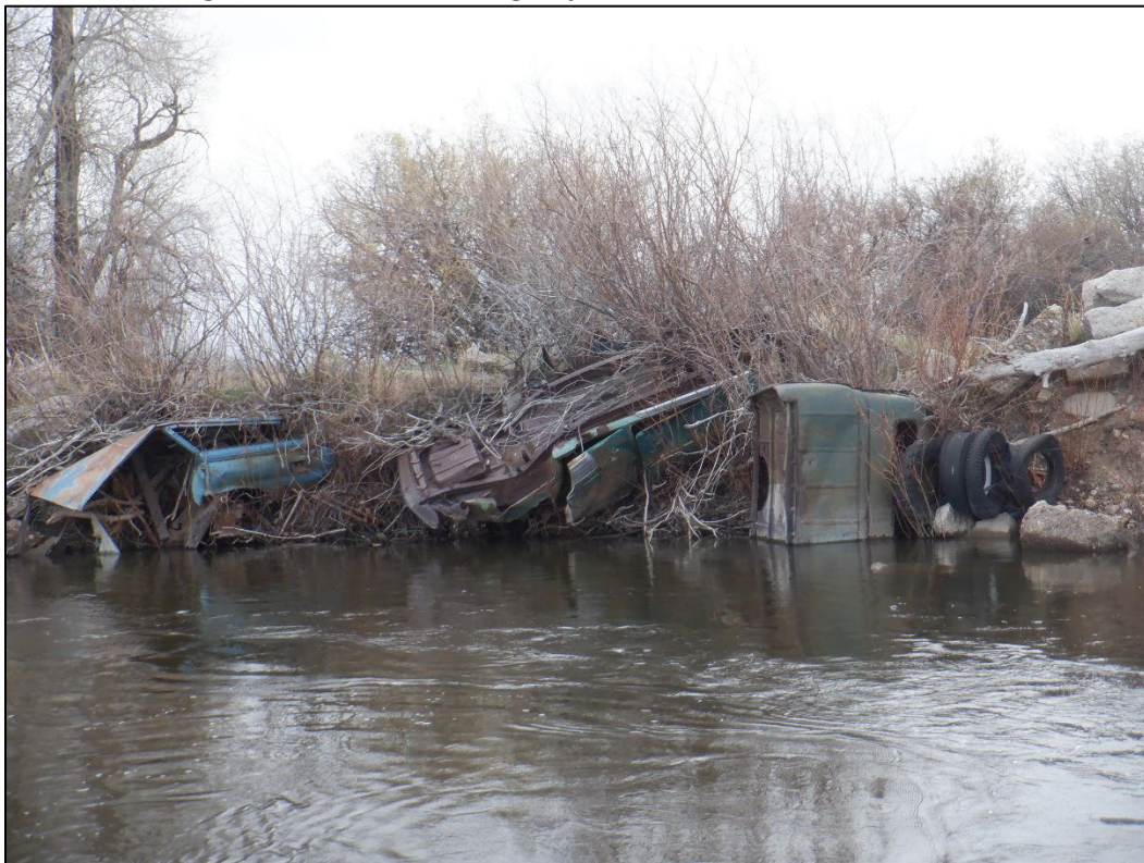
Figure A-6. Bank armoring with old automobiles and other trash.
