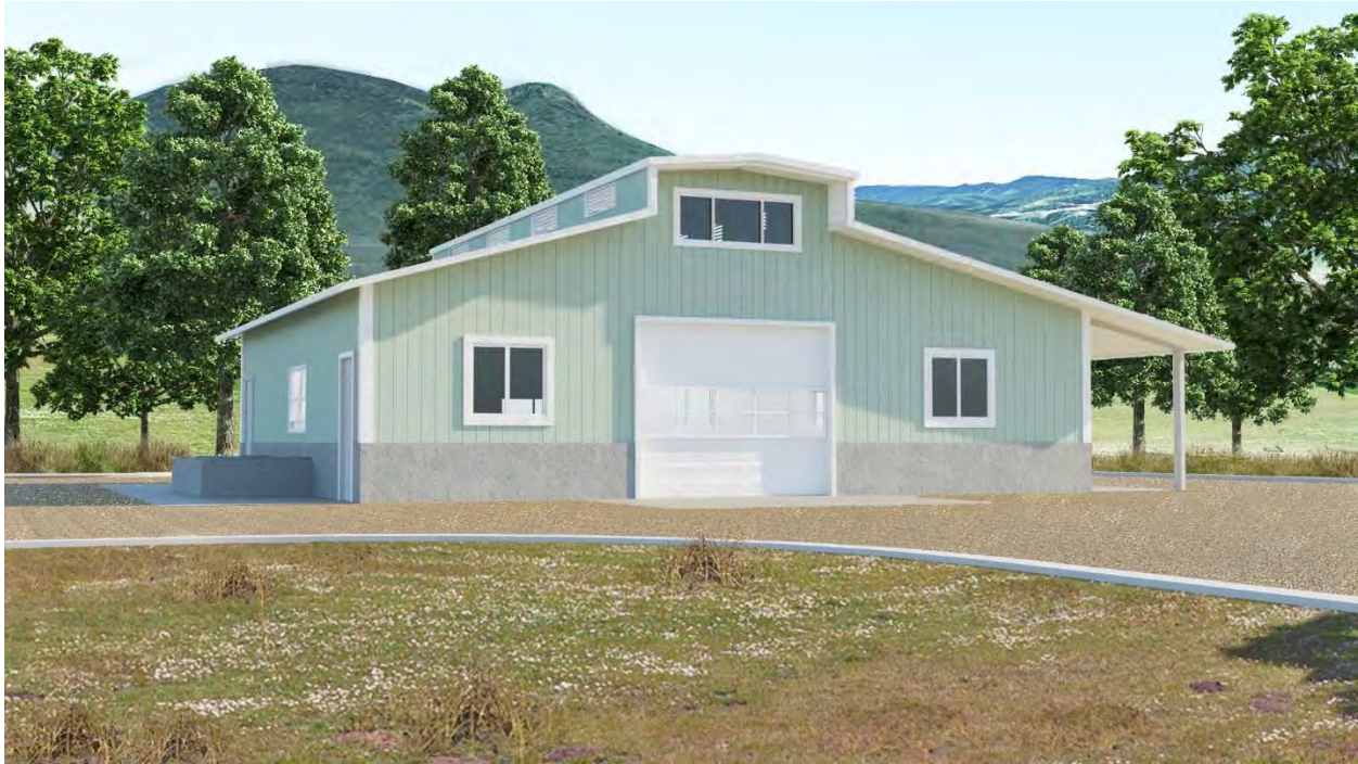
Figure 24: WWTP Building with Driveway
