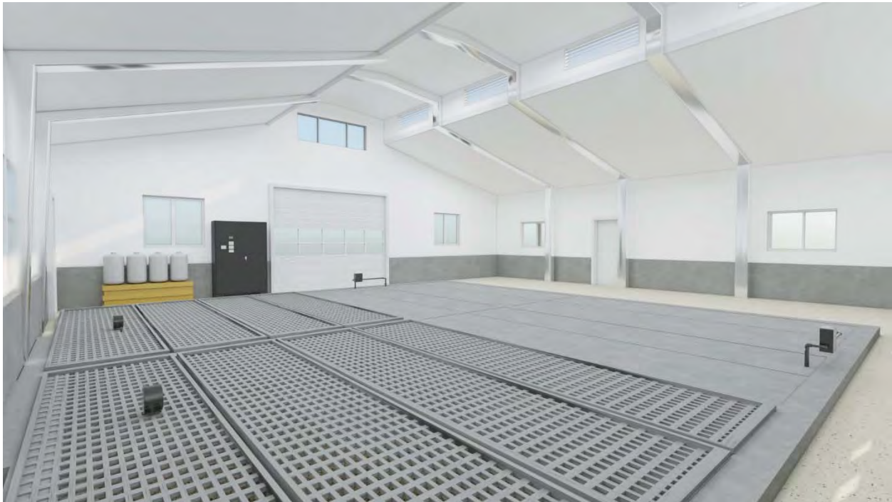
Figure 19: All Process Tanks are Indoors Except the Chlorine Contact Tank
