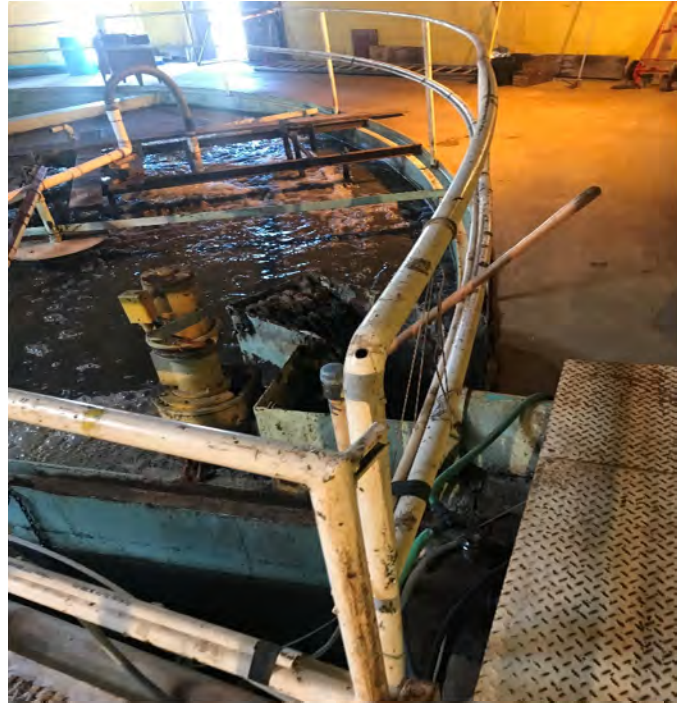
Figure 3: Photo Existing Facility
