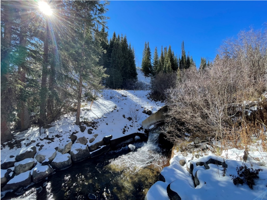
Coal Creek - Proposed Site Location
